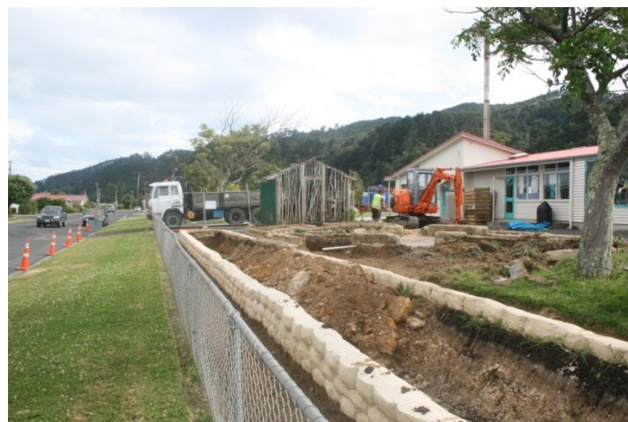
Excavating the gardens
